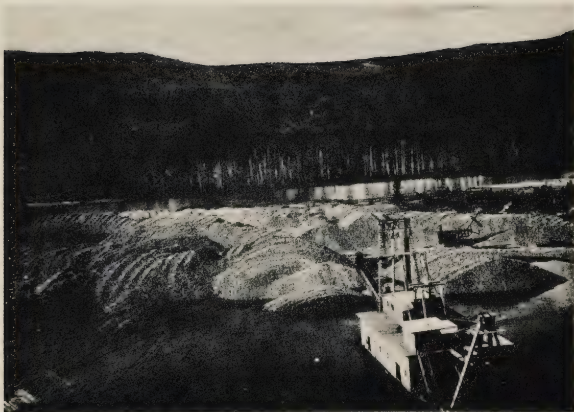
Dredge at work.
